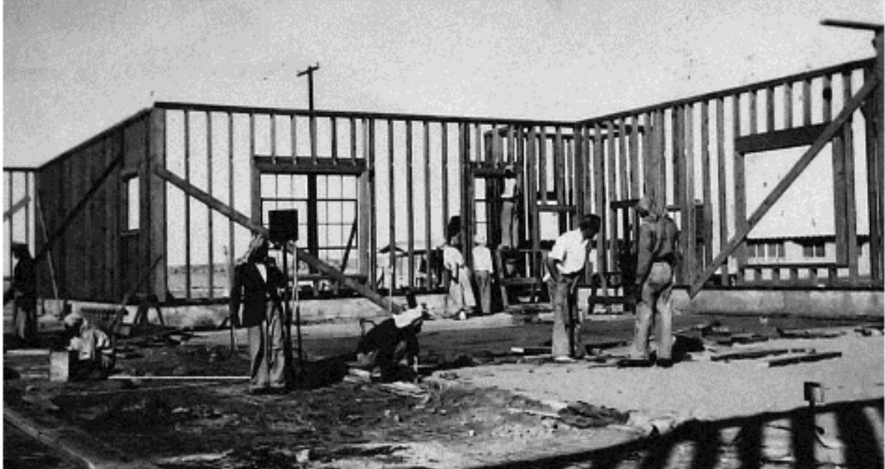
Figure 1.2: Timber frame construction at the Dhahran camp, 1936. Photographer unknown. Courtesy of UC Santa Barbara Library, Saudi Arabia Oil Photograph collection, Bernath Mss 366 as located in “Oil + Architecture,” Alshabib and Ridgway.
