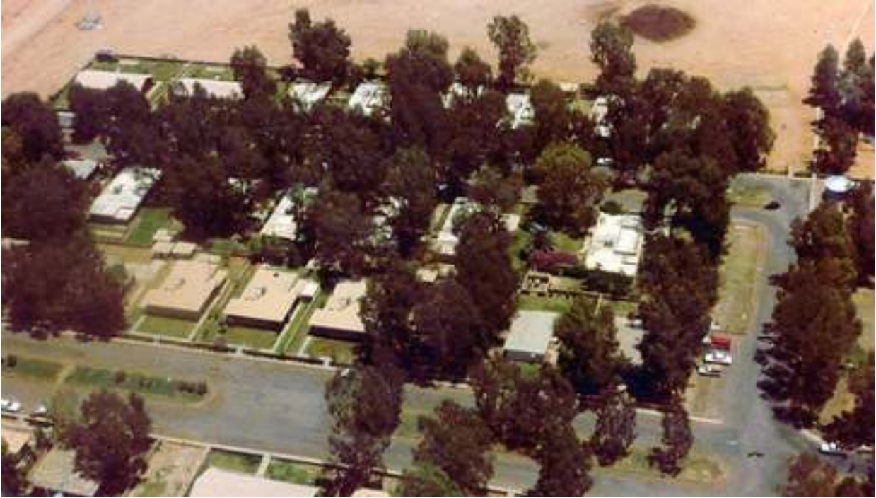
Figure 1.13: Housing for Saudi Aramco employees. Note the homes positioned in the center of the lots with no inner courtyard, ca. 1979. Courtesy of AramcoWorld.
