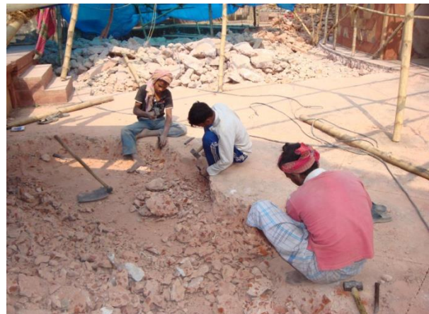
Concrete removal on terrace. Source : "Humayun's Tomb Complex Restoration | Plan | Archnet."
