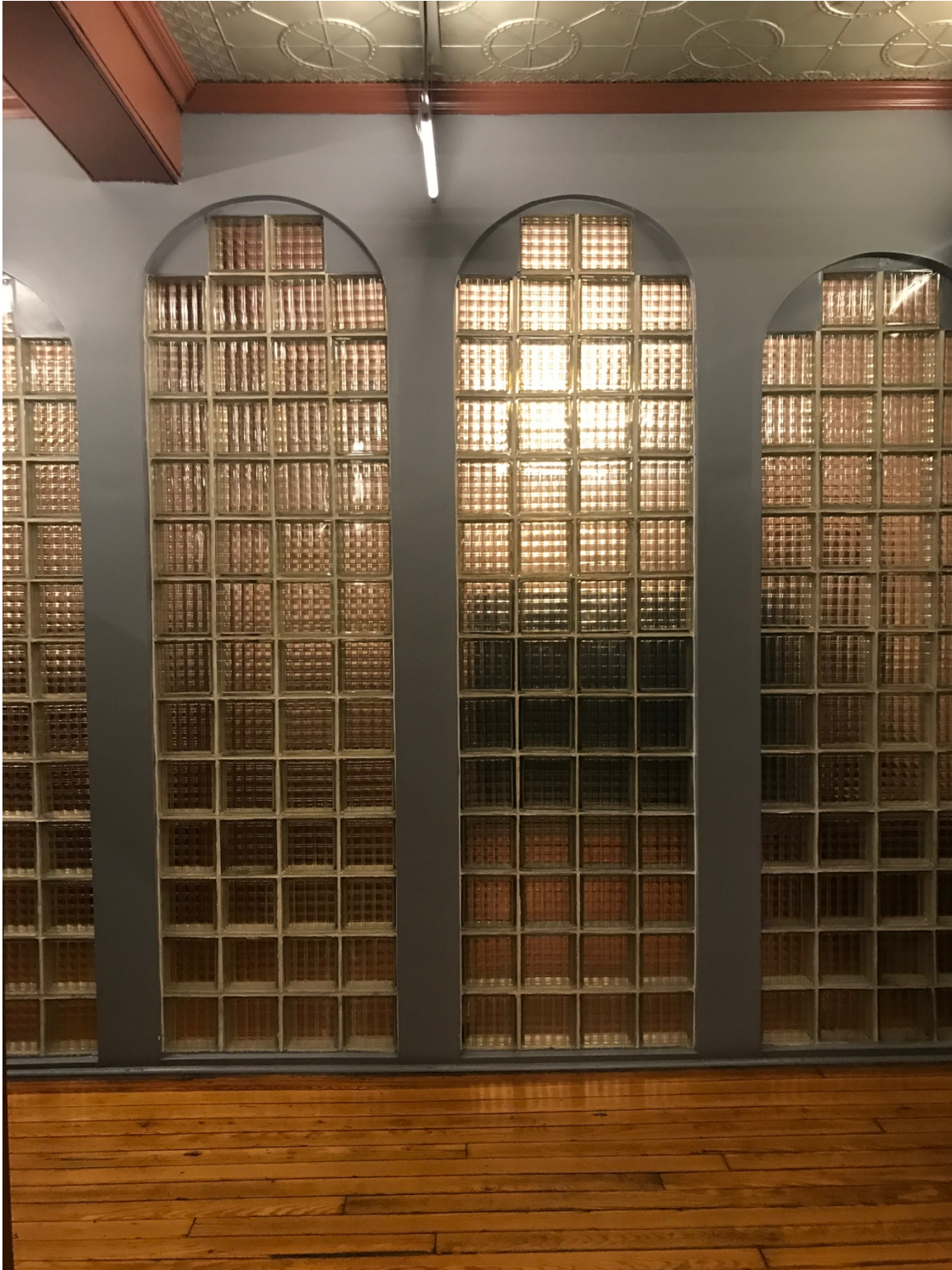
Figure 12 Museum wall constructed of glass blocks from east window Source: Emily Kahn, December 2019
