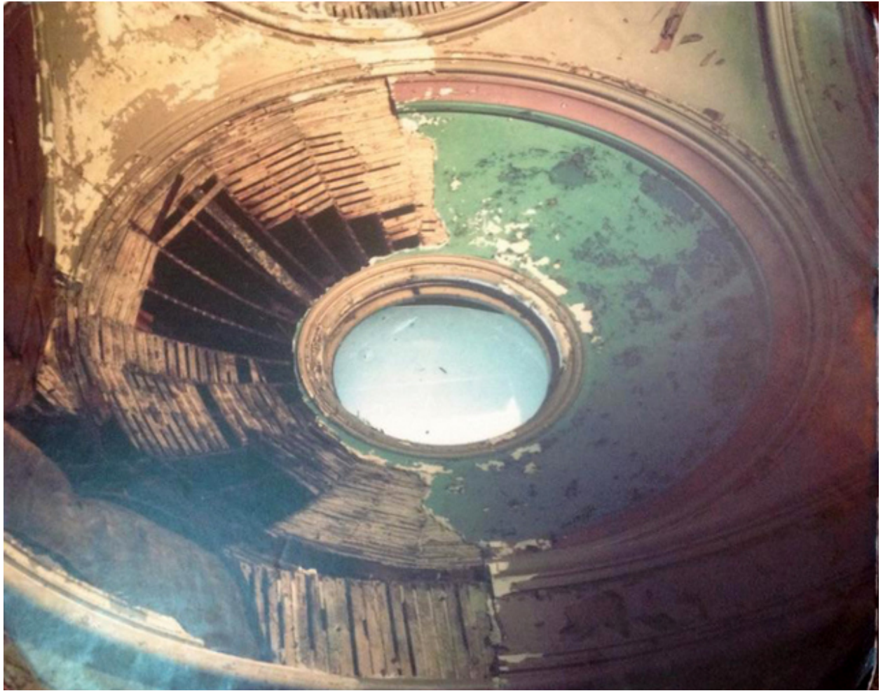
Figure 2 Decayed paint, lath, and plaster in dome above Women's Gallery
