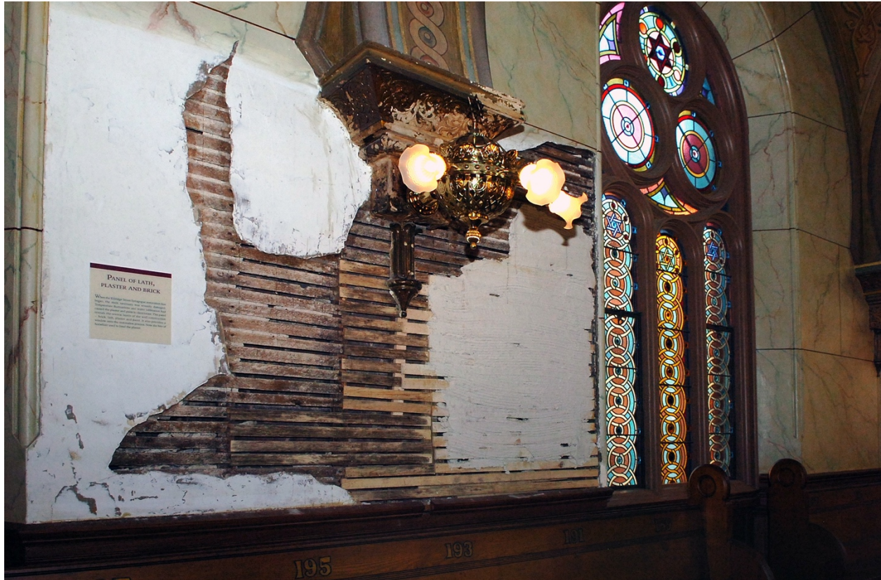
Figure 8 Exposed lath and plaster in restored synagogue
