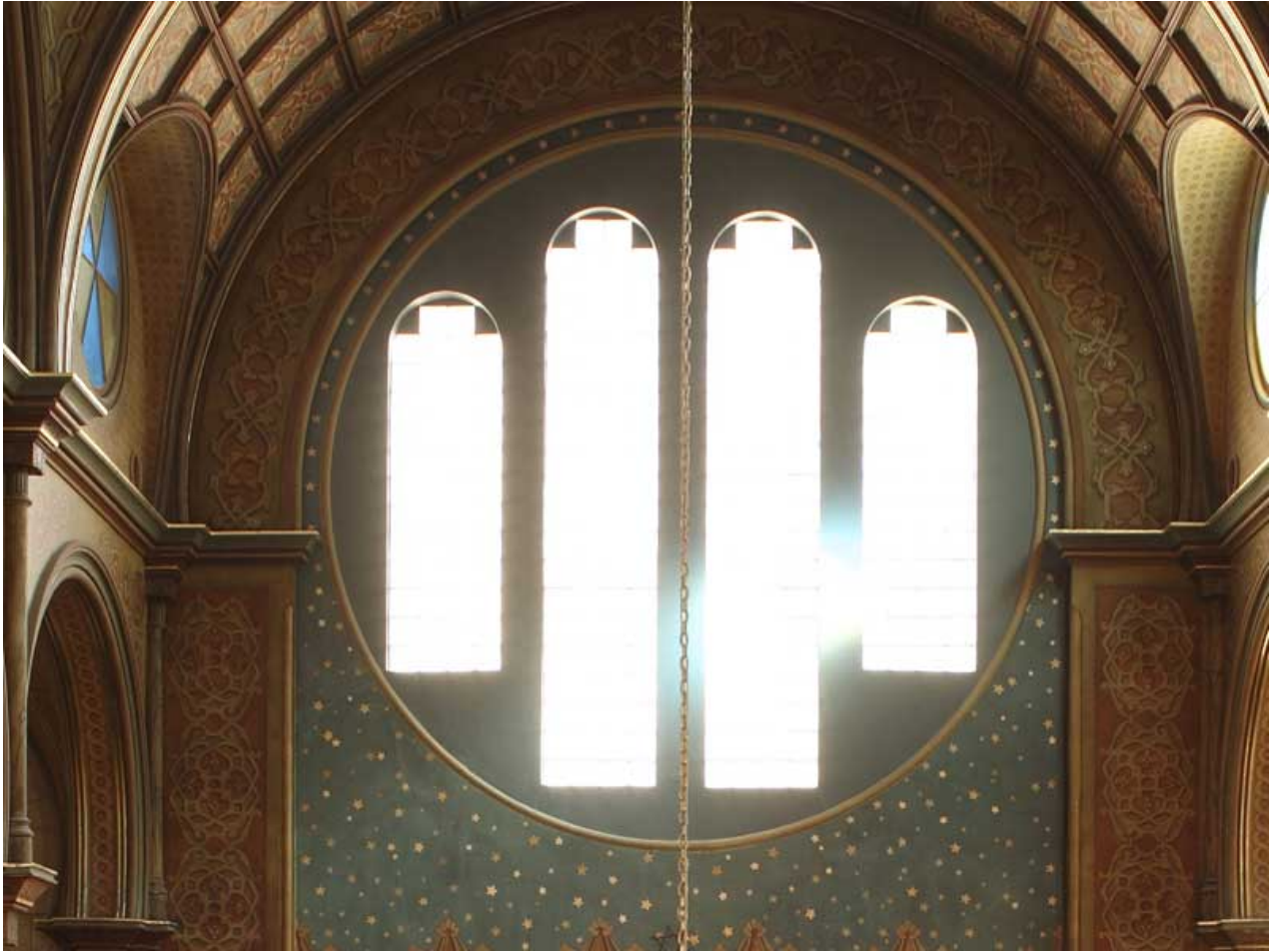
Figure 9 Glass blocks in the shape of tablets infill east window pre-restoration
